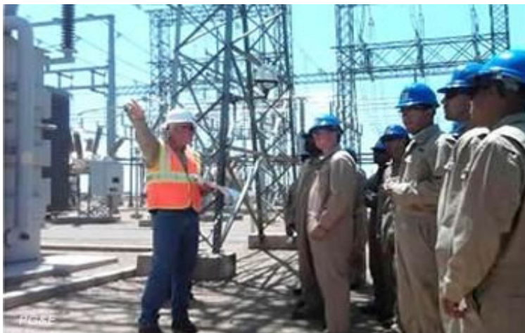
McCall substation tour
