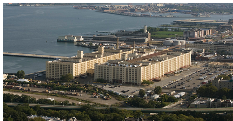
Built in 1919, Brooklyn Army Terminal in Sunset Park, Brooklyn is now home to over 100 companies in diverse industries such as bioscience, food, fashion and electronics.
