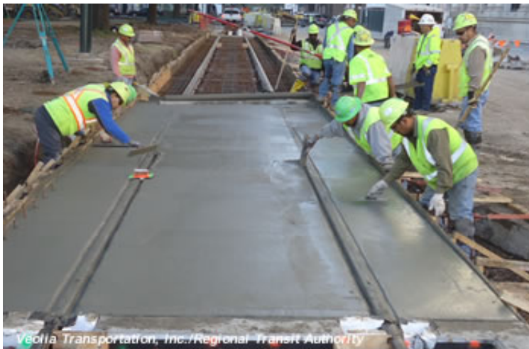
Workers place concrete for new track.
